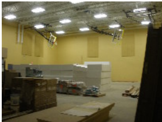
Building Addition – New Gym, Current Material Storage Area
