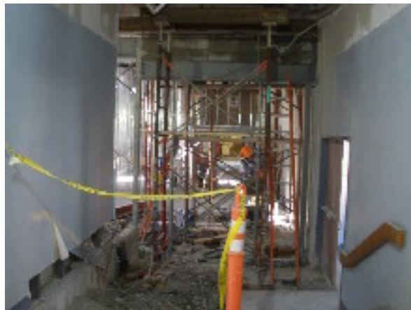
Corridor Renovation – Future Ramp Location
