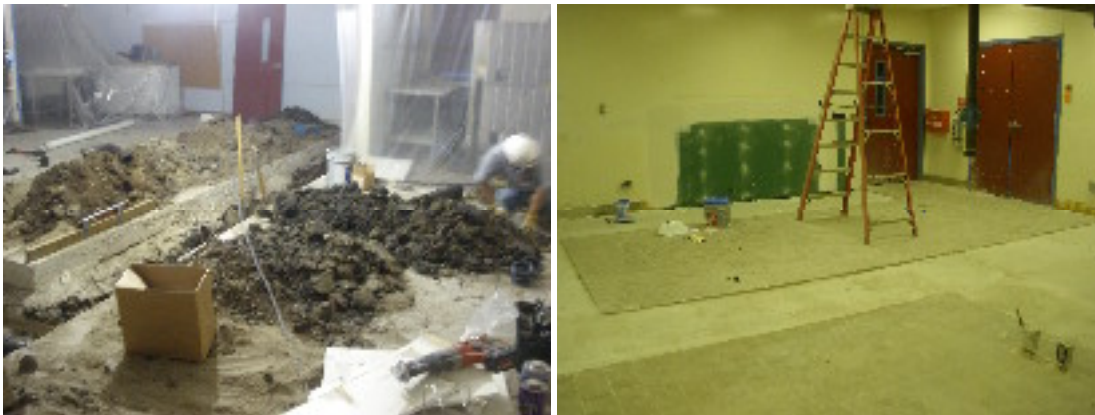
Kitchen Renovation (Left-During Underground Work, Right-Patching)
